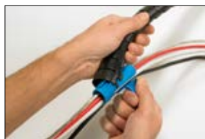
Place the HAT applicator tool in one end of the Helawrap cable cover.
