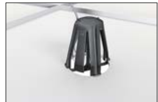
2. Push the spikes into the plasterboard to prevent shifting and disconnect the tool.
