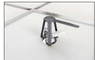
3. Install the downlight.
