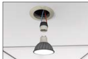
3. Connect the bulb to the socket and lock into the correct position.
