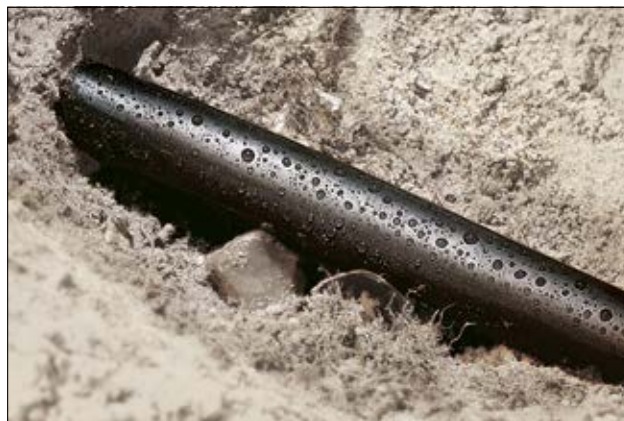
TREDUX HA47 - application below ground.
