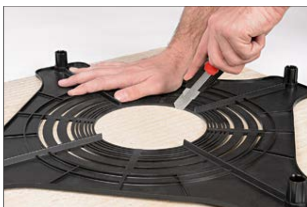
Use the SpotClip-Plate as a stencil to cut the fixing hole into the ceiling plate.
