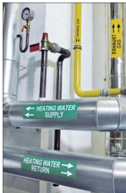
Large and highly visible pipe marking.
