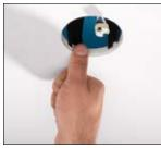
2. Push the spikes into the plasterboard to prevent shifting.
