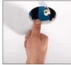
3. Push the spikes into the plasterboard to prevent shifting.
