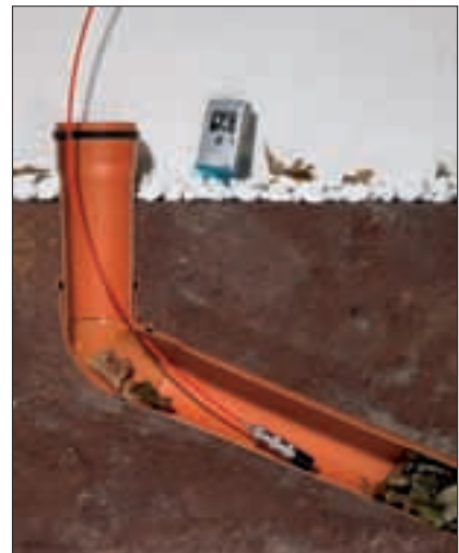
The camera can be used to detect duct blockings.
