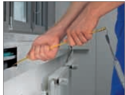
Installing cables through trunking. No problem with Cable Rod.
