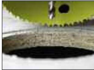
A 2mm rebate is length which allows the cover plates to be installed flush with the existing floor
